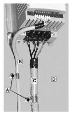
Installation: Shielded cable must be used for all control and power cables and exposed wiring must be kept as short as possible. The figure to the right shows the control cable (B) and motor cable (C) with the shield grounded with clamps (A) to a grounded, electrically conductive mounting panel (D). The motor cable must be of a low capacitance specification:
